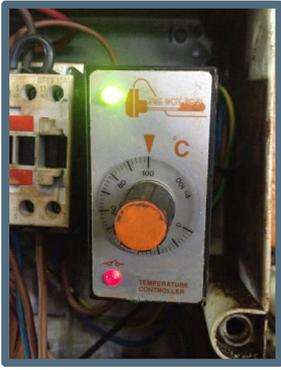
The temperature profile of the plating tanks is also far more stable with auto control than without it. When operating on auto control, the variance is as low as 1.2 ° C while without auto control the temperature has a wide range of 7.6 ° C.
